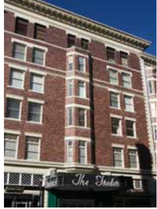
8 HOTEL FREDERICK BUILDING 940 4th Avenue
