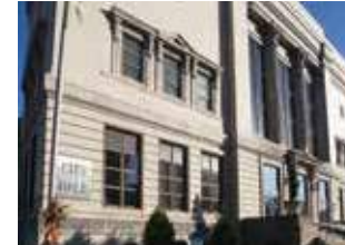
12 HUNTINGTON CITY HALL 800 5th Avenue
